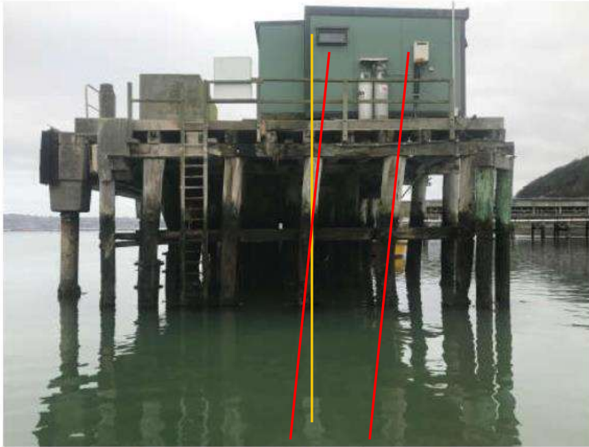
Photograph 1 – End of Wharf looking South.
